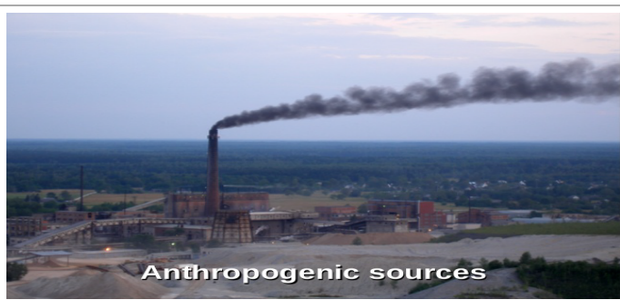
Figure 5: Shows the example of arsenic disposal in air
